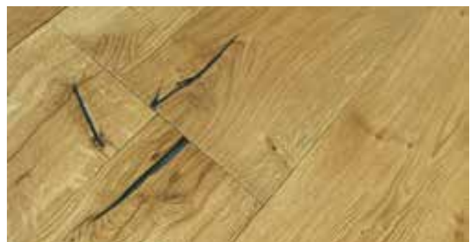
Detail: Cracks Eiche Windsor
